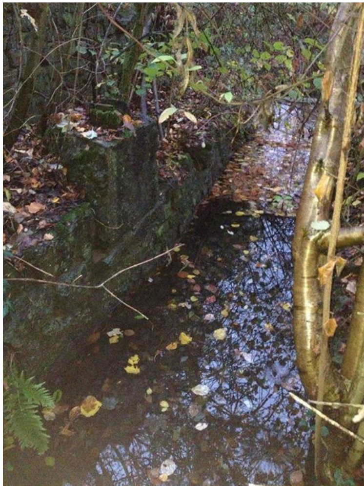
Another view of where the water wheel was located, with the mill race ditch below. The water was diverted from the river a half kilometer or so upstream so that it came out at the top of a wall that is behind me in this picture. There would have been a wooden trough coming out from the ditch at the top of that wall to a spot above the wheel, enabling it to turn.
